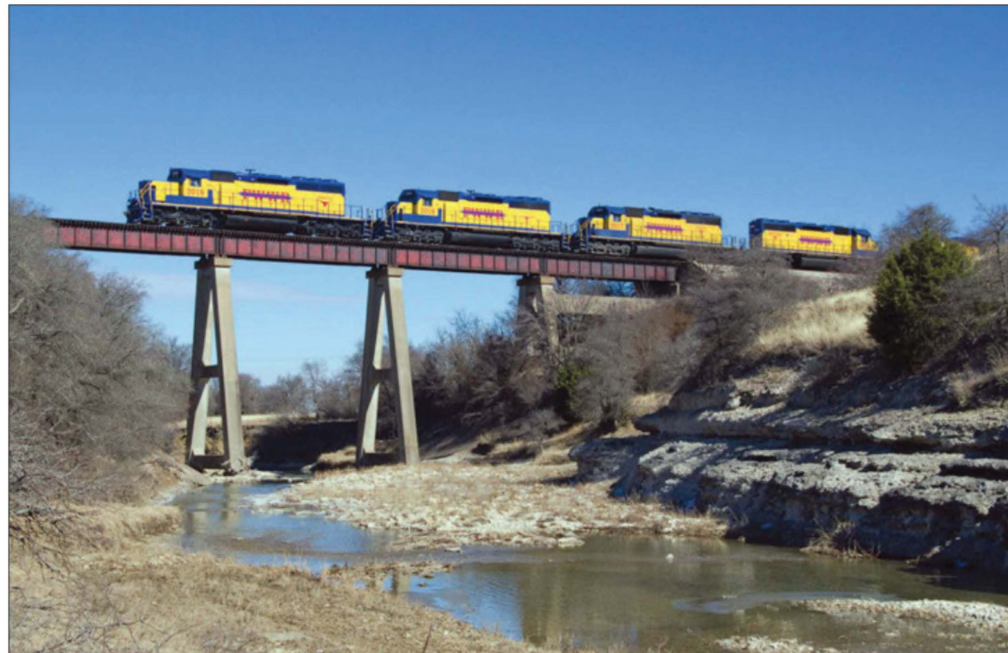
ABOVE: All four of the road's six-axle units soar above Mustang Creek with a heavy FWDU train on February 6, 2011. Concrete piers support the 250-foot long deck girder bridge. LEFT: On March 3, 2011, Job 402 passes the former Santa Fe brick station at Comanche. This location also sports one of the few Santa Fe-era station signs remaining along the line.
