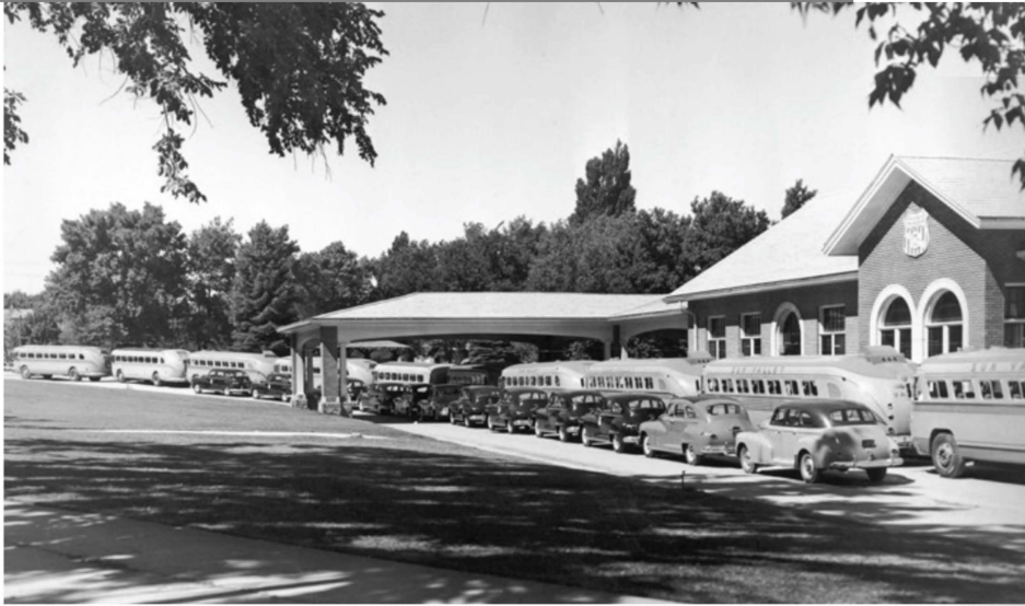
ABOVE: A line of buses and cars at Cedar City. Based on the shadows, the Utah Parks Special is about to arrive. The buses are lettered for Sun Valley, another UP venture that needed buses in the winter for the arriving skiers. The railroad maximized the vehicles' utilization by moving them among its tourist destinations. SOUTHERN UTAH UNIVERSITY
