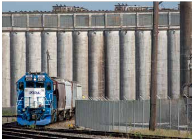
Chemicals may be king on the PTRA, but the railroad also handles intermodal traffic and a seasonal burst of grain.
