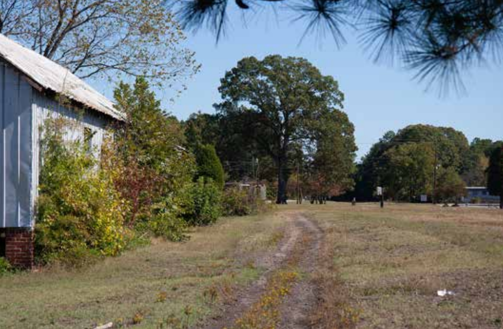
The goal of rebuilding the Seaboard S Line seemed very far away when this photo was taken at Norlina, N.C., in October 2007. A structure once used for maintenance still stood but the right-of-way was no longer visible. Norlina is the place where the now-abandoned branch to Newport News, Va., once diverged. Two photos, Bob Johnston
