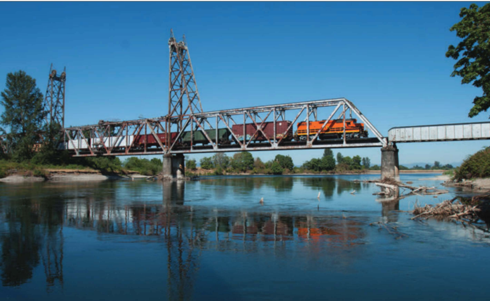
BELOW: The northbound American Turn glides over the rolling waters of the Willamette River between Junction City and Harrisburg on July 31, 2008. Built in 1910 by Waddell & Harrington, the vertical lift was used only briefly and the river has since changed course to flow under a fixed span.
