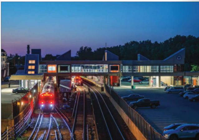
RIGHT: It's twilight time at Oak Grove station at the northern end of the Orange Line in Malden. Oak Grove opened as the northernmost stop on the rebuilt northern portion of the Orange Line on March 21, 1977. The low geometric design of the station is a common element of the Haymarket North Extension stations. MBTA later added new elevators to all the stations for improved ADA accessibility.
