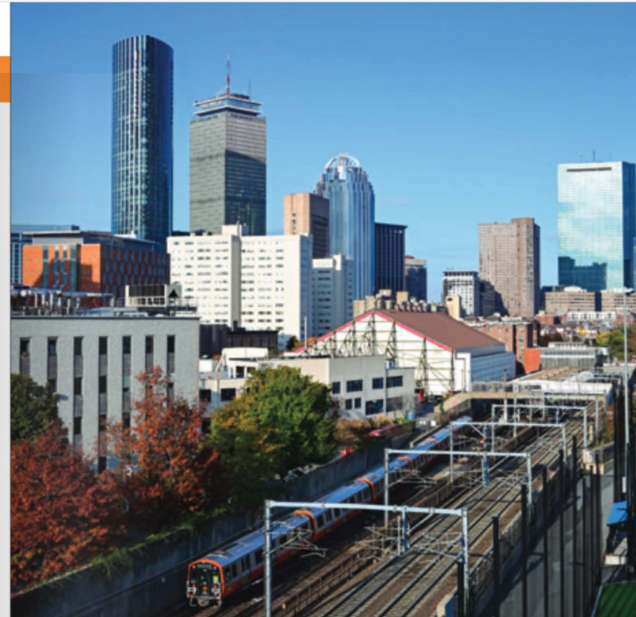
LEFT: Boston's Back Bay skyline looms over the Southwest Corridor's five-track right-of-way on November 5, 2023. The three nearest tracks are shared by Amtrak and MBTA commuter rail trains, and the two farthest are the Orange Line tracks to and from Forest Hills.
