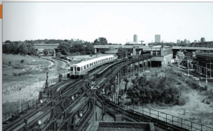
LEFT: In a 1982 image taken from the roof of Tower H just beyond the old Forest Hills terminal of the Washington Street Elevated, a nearly new train of Hawker-Siddeley cars approaches the storage yards to the south. The cleared area on the left is the former New Haven main line where the Southwest Corridor trench and new Forest Hills station will be built. RICHARD CHEEK PHOTO, LIBRARY OF CONGRESS HAER MASS,13-BOST, 127-82
