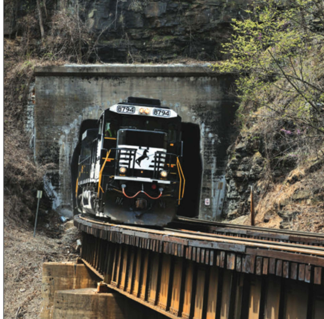
LEFT: With four standard-cab GEs leading the charge, eastbound loaded Virginia Power coal Train 838 emerges from Laurel Tunnel and crosses Tug Fork on April 19, 2014. The tunnel clearances were enlarged in 2009 as part of the Heartland Corridor project. This location is right off U.S. Route 52 between Roderfield and Iaeger, W.Va.
