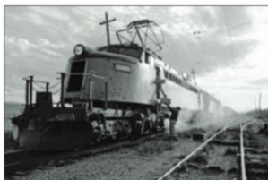
ABOVE: On June 10, 1974, after running 25 miles from Lenep to Two Dot, Mont., with a defective traction motor on E-77, the engineer and head brakeman on Train 264 poured water on the journal of the smoking motor. This proved futile and the crew are unloading their grips before they set out the Joe.
