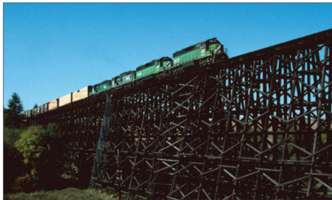
RIGHT: Eastbound Burlington Northern Train 398 (Albany-Pasco) crosses the big trestle over Dick Road just east of Bowers, Ore., in October 1986. RANDY NELSON. BELOW: The speed is down to under ten m.p.h. as a loaded Harbor Turn crosses the Holcomb Creek trestle with a Geep and SD45 on June 17, 2011. This impressive bridge is set on a 1 percent grade, and the train is struggling to maintain speed. ROBERT W. SCOTT
