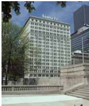
Santa Fe’s headquarters on Michigan Avenue. David P. Oroszi
