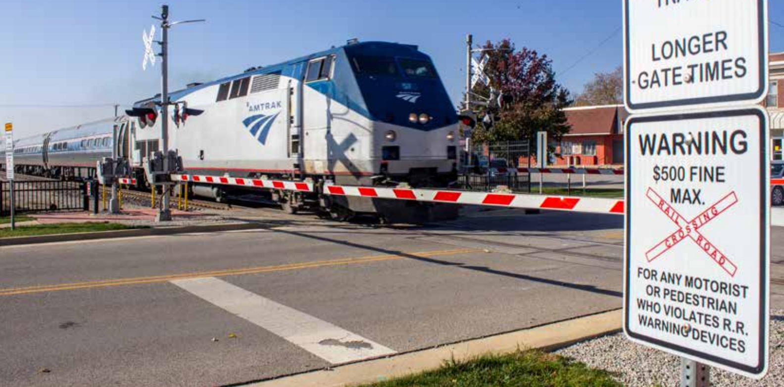
Four-quadrant gates, closed-corridor fencing, and additional signage warning of "longer gate times" protect a grade crossing in downtown Odell as Lincoln Service train No. 302 passes on Nov. 16, 2016. Two photos, Bob Johnston
