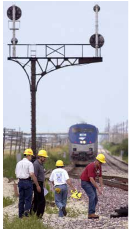
Amtrak and Union Pacific personnel look over a switch at Ballard, Ill., during test runs of equipment involved in the 110-mph program in July 2002. Steve Smedley
