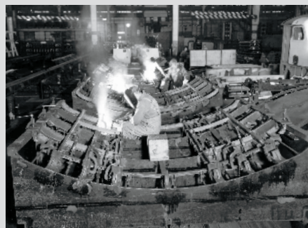
6 Work on the roof was begun inverted, with parts held in fixtures for welding.
