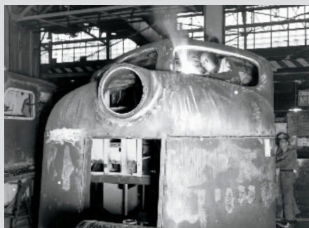
5 After the welded-up cab frame was plated, the welds were ground down.
