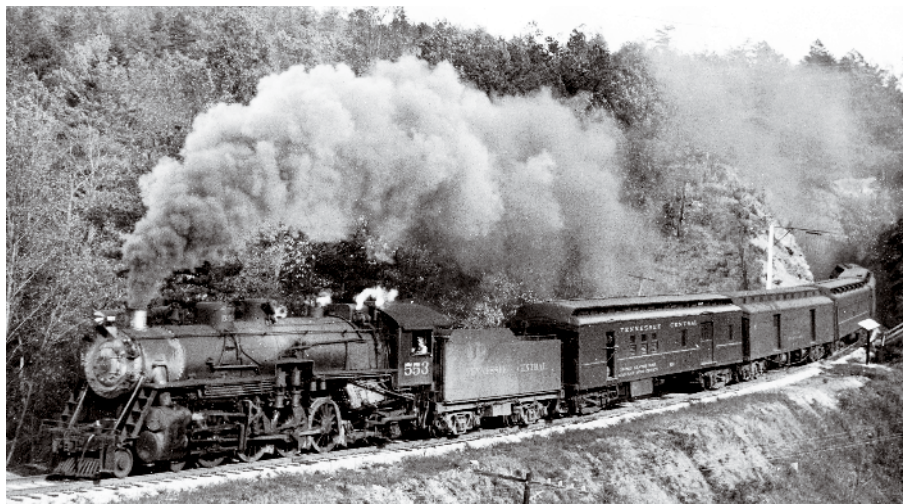
Tennessee Central's only tunnel, through Walden's Ridge 3 miles west of Rockwood, has just seen the passage of Harriman–Nashville train 1, behind 4-8-2 No. 553, in November 1947.
