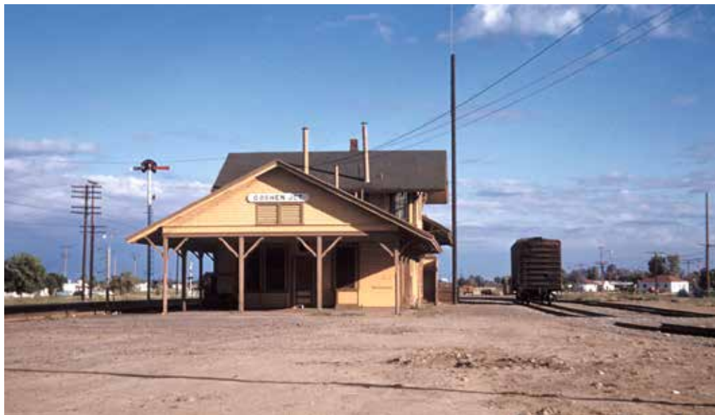
The station at Goshen Junction hadn’t changed much between author Read’s time there as a telegrapher in the mid-’50s and April 19, 1962, when this southward-facing photo was made.
