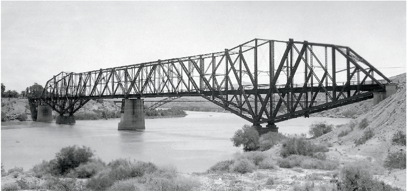
The 1890-vintage gantlet-track bridge over the Colorado River at Topock, Ariz. (above), was a bottleneck for all Santa Fe traffic moving in and out of California. The double-track replacement that opened in 1944 (right, in a 1953 photo) was on a new alignment that dispensed with a number of sharp curves.
