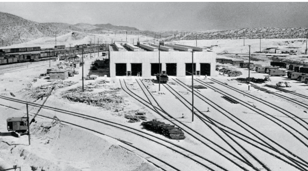
The Santa Fe converted several stalls in the roundhouse at Winslow, Ariz. (top), for FT servicing. The steam facility was ill-suited to diesel work, and the lessons learned from it resulted in a completely different design for the new diesel house at Barstow, Calif. (above).
