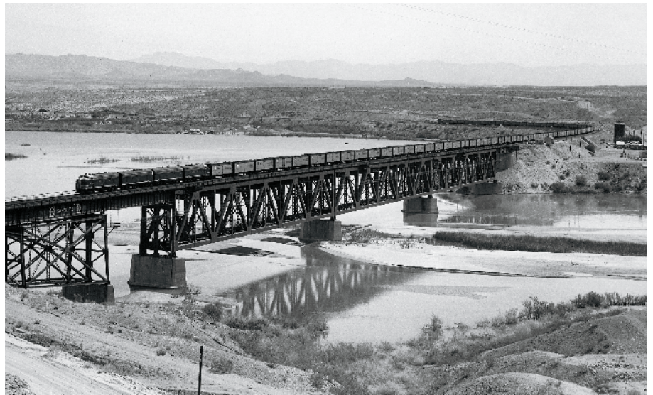
The 1890-vintage gantlet-track bridge over the Colorado River at Topock, Ariz. (above), was a bottleneck for all Santa Fe traffic moving in and out of California. The double-track replacement that opened in 1944 (right, in a 1953 photo) was on a new alignment that dispensed with a number of sharp curves.
