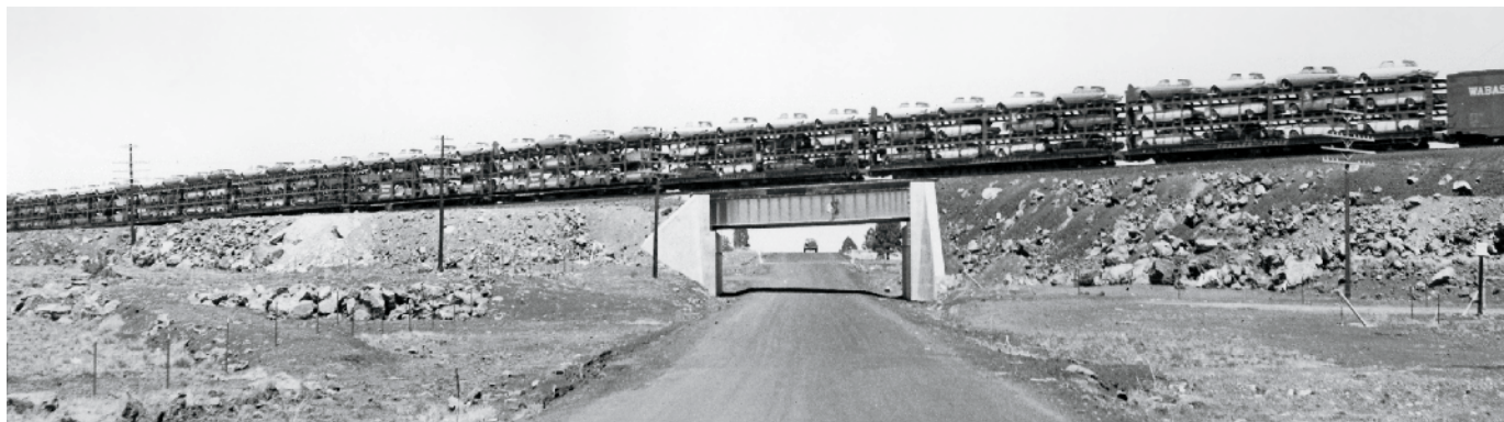
State-of-the-art railroading, circa 1961: Modern tri-level auto-racks sail along a fill and over a local road on the new line north of Williams.
