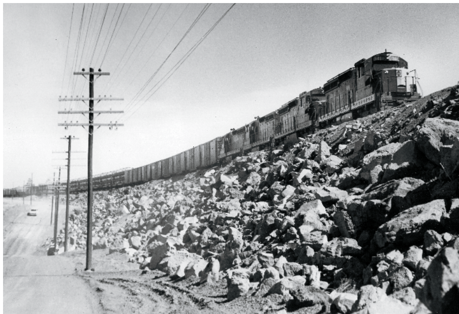
An SD24 quartet rides over a rock fill typical of those found throughout the new alignment.
