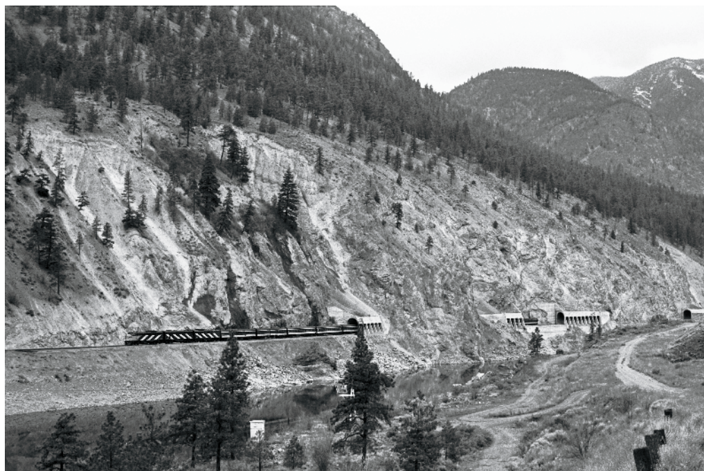
A westbound Super threads through Snoonka Tunnels along the Thompson River in British Columbia on April 13, 1975. To navigate the steep, unstable cliffs, Canadian National built three tunnels and four rock sheds totaling 1,750 feet in a stretch of only 2,112 feet of track.
