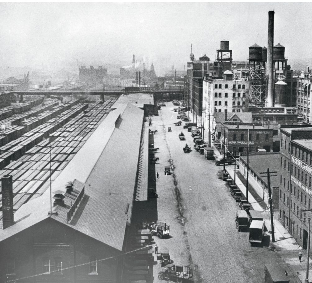
In the 1920s, long before superhighways and 53-foot semi-trailers, cities were almost completely dependent on railroads for their needs. Here, boxcars jam the tracks at the Milwaukee Road’s downtown freight house on Fowler Street (now St. Paul Avenue) in Milwaukee.
