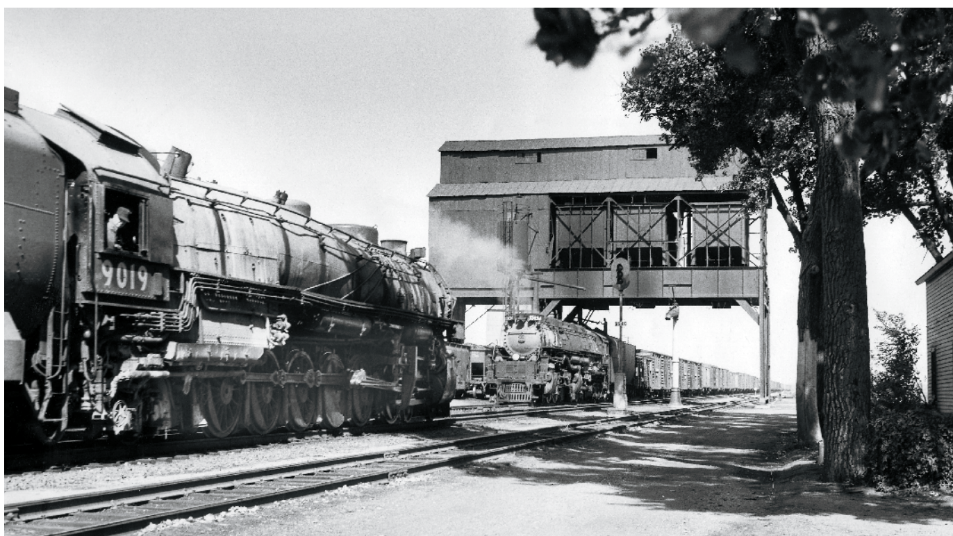
OGALLALA, NEBRASKA: The engineer of UP three-cylinder 4-12-2 9019 glances back at the photographer as he eases an eastbound freight up to the mainline coaling stage at Ogallala, 51 miles west of North Platte, in mid-1949. Ahead, the fireman of Extra 3934 West finishes fueling his 4-6-6-4 Challenger.
