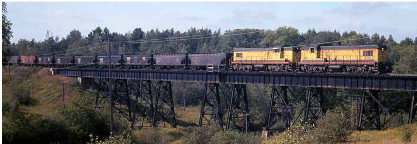
Having just left Ewen, Mich., AS616s 210 and 204, their lettering intact despite the 1960 Soo merger, lead Superior–Marquette train 22 across the Baltimore River west of Bruce Crossing September 3, 1961. Heavy freights were handled by 12 C-C Baldwins like these, plus 4 center-cabs.
