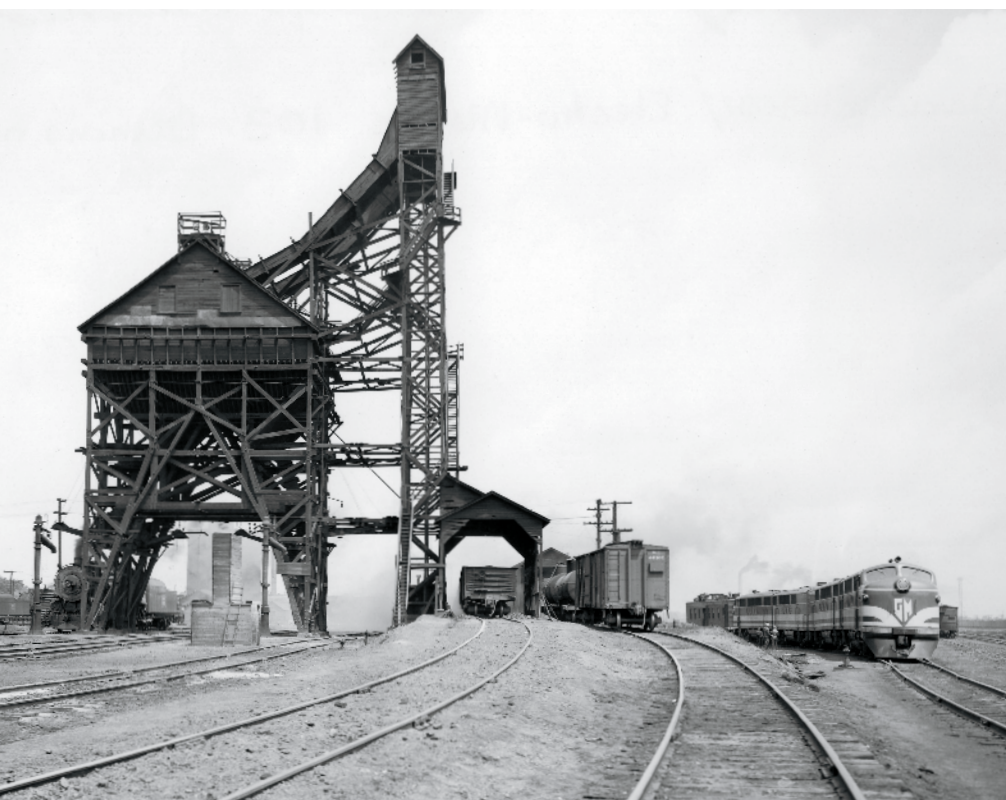
No. 103 is dwarfed by a coaling tower at the Rock Island's Blue Island Yard outside Chicago. The FT and its successors would end the need for such costly infrastructure. CLASSIC TRAINS coll.
