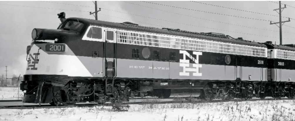
The first two of New Haven's dual-power FL9s were built with Blomberg front trucks, which were soon replaced by Flexicoils with third-rail shoes. In the cab, extra controls and instrumentation were required for straight-electric operation. The 60 FL9s were NH's only F units. EMD
