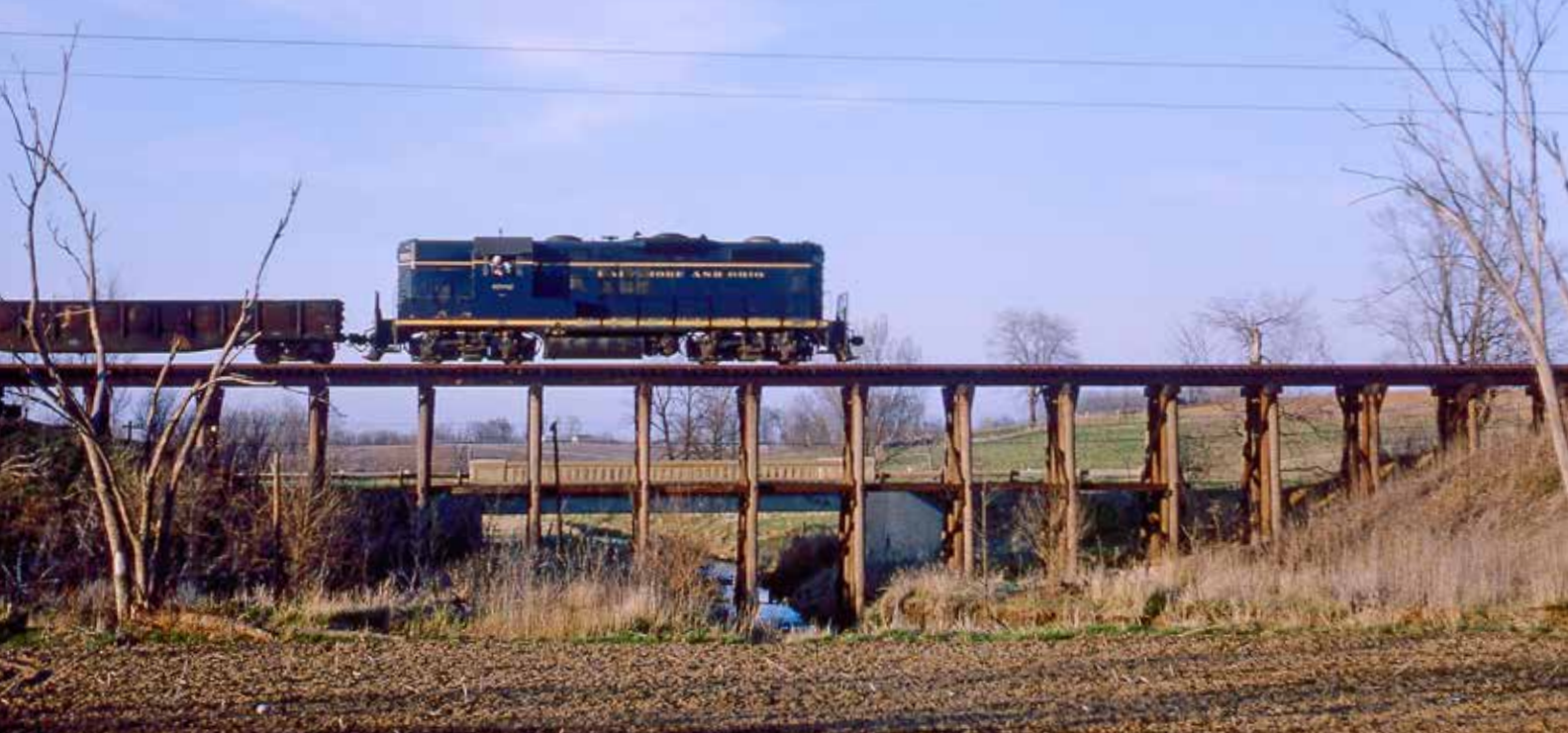
This trestle east of Pleasant Plains, crossed by GP9 6592 with the eastbound local on April 19, 1965, makes obvious why Geeps were the heaviest power allowed on the line. Visible beyond is the Highway 125 bridge.
