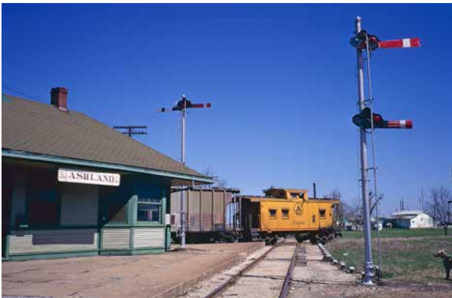
Caboose C2040 on the westbound local of April 4, 1973, crosses ICG's "Jack Line" at Ashland. In years past, the joint depot included a two-story interlocking tower facing the diamond.
