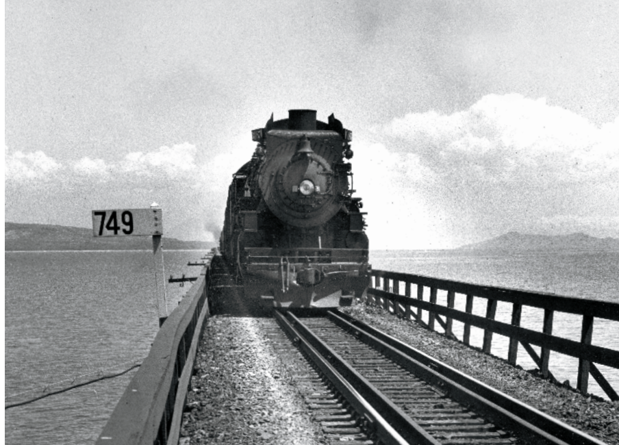
Southern Pacific's 103-mile Lucin Cut-off opened in 1904 to replace the 1869 line via Promontory Summit, Utah. It included 27 miles of fill and trestle across the Great Salt Lake. SP
