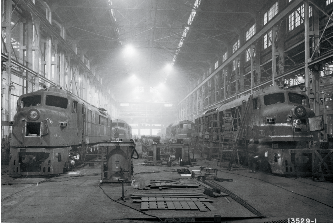
Baldwin's smoky, steam-era shop at Eddystone, Pa., hosts mammoth 2-D+D-2 "Centipede" passenger diesels in the late 1940s. Baldwin
