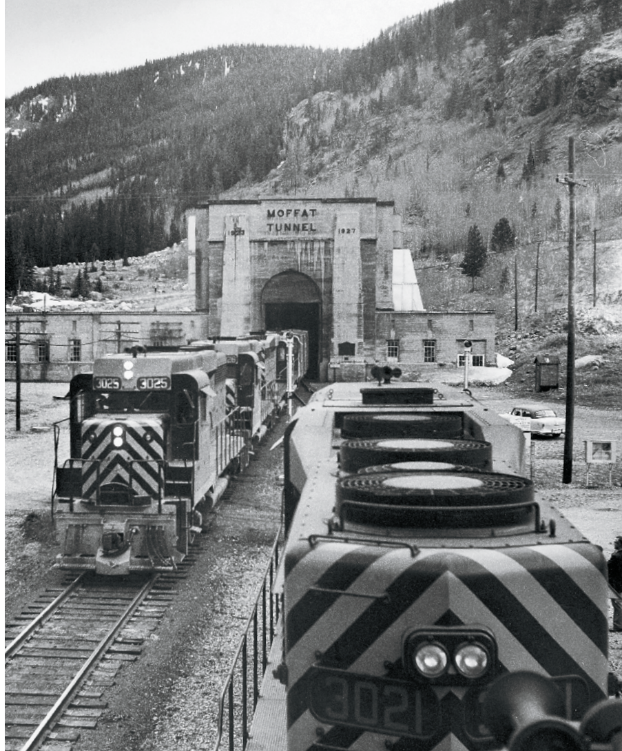
Brand-new Rio Grande GP30s meet at the east portal of the 1928 Moffat Tunnel, which, with the 1934 Dotsero Cutoff, gave Denver a connecting rail route to the west. Bruce R. Meyer
