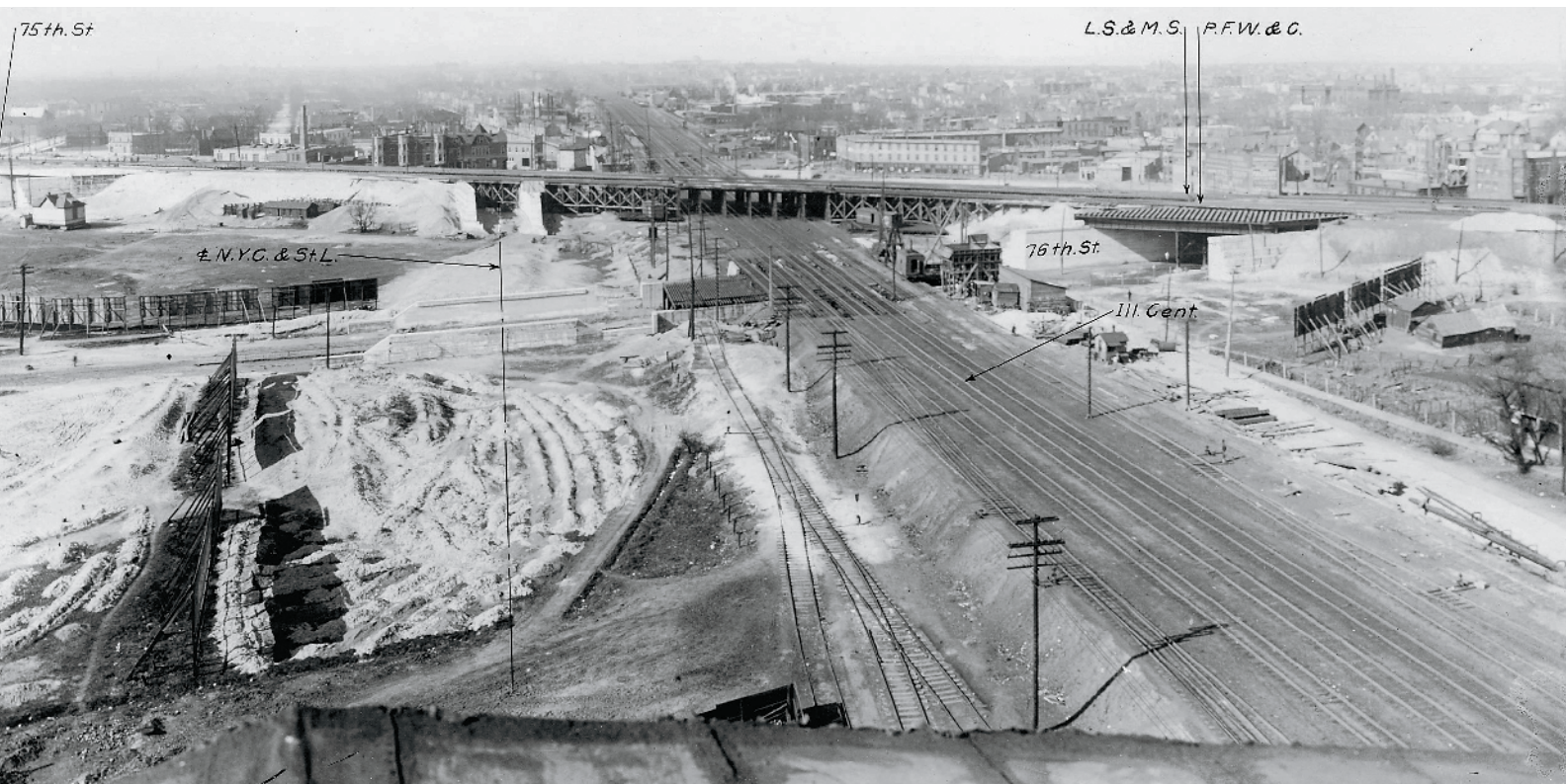
Driven by cities desiring to eliminate grade crossings, and by their own quest for efficiency, railroads did major grade separation work in the early 20th century. Chicago's Grand Crossing project, seen in 1912, eliminated dozens of street crossings and diamonds. John Gruber collection
