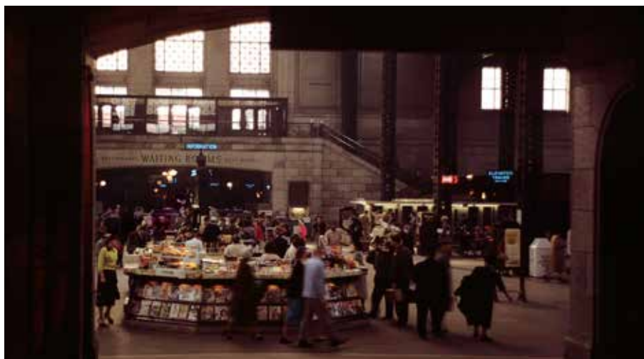
Opened in 1925, Union Station was the biggest and last-built of Chicago's six mainline terminals. The concourse, seen here, was razed in 1969; the waiting room survives. Linn H. Westcott
