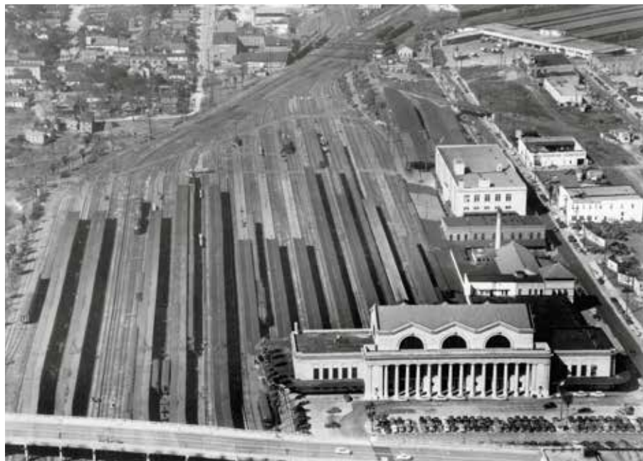
Jacksonville Terminal, rail gateway to Florida, got a new, classically styled head building in 1919. Other improvements gave it a total of 11 through and 15 stub tracks. Jacksonville Terminal Co.
