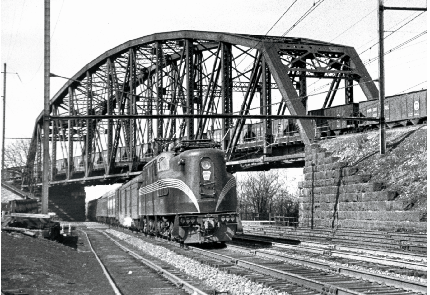
In the 1890s and 1900s, the Pennsylvania built low-grade lines that separated freight and passenger traffic, followed by electrification in the 1920s and '30s. At Whitford, Pa., in the early '50s, a G1 speeds the Admiral east beneath the Philadelphia & Thorndale freight line. David G. Knox
