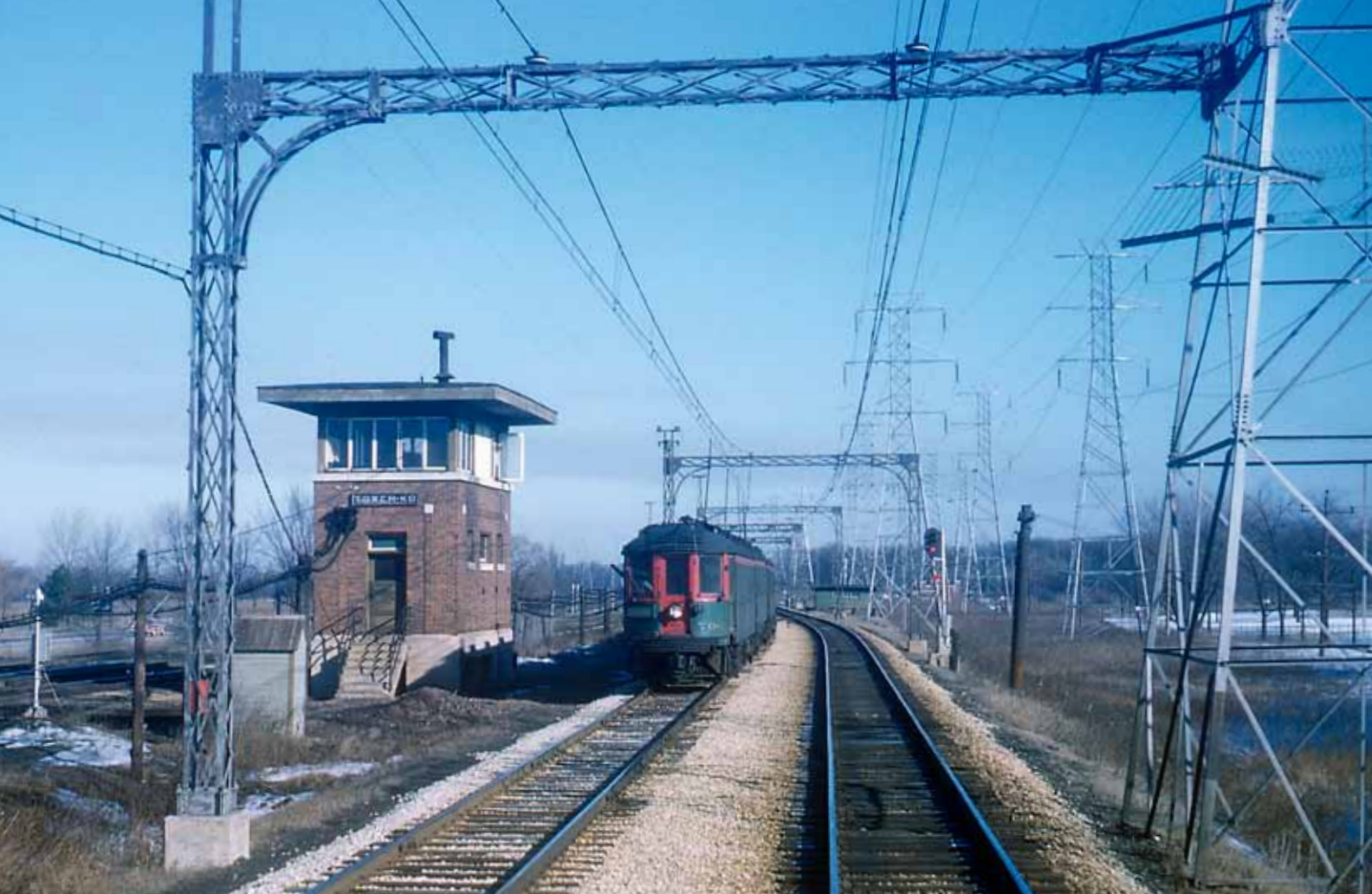
Seen from the front of a northbound train, a train to Chicago passes KO Tower in Lake Forest, where the Skokie Valley Route crossed a C&NW line, on February 23, 1959.
