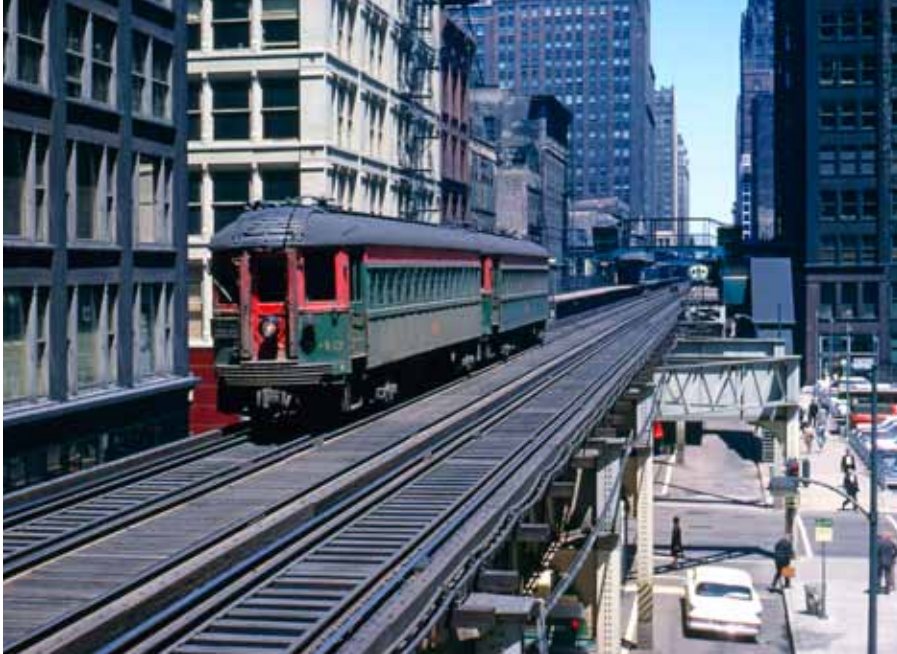
On the west side of Chicago's Loop, an inbound North Shore train approaches the Quincy & Wells elevated station on June 13, 1962. In the distance—and also approaching—is a CTA "L" train, both Loop tracks being operated in a one-way, counterclockwise pattern at the time.
