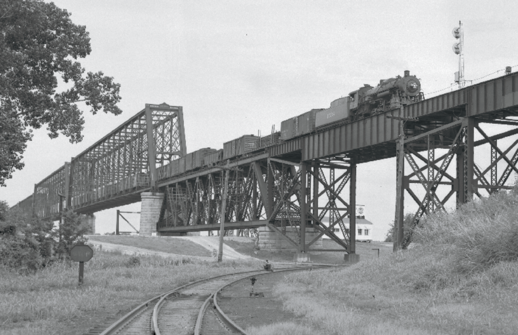
Mikado 1538 leads a northbound off the Cairo side of the bridge June 20, 1950. All of the steel trestlework between the through truss spans and the embankment to the right were replaced in 1934. By the time of this photo, crews were replacing the nine spans of the superstructure.
