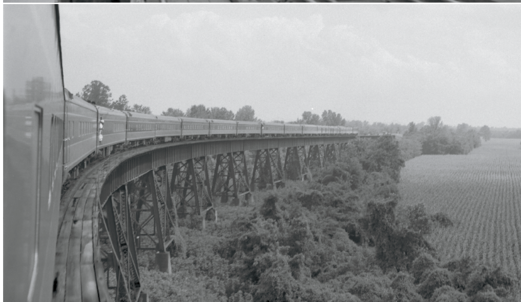
Under gray skies on December 2, 1951 (top), an E7 leads a southbound passenger train onto the bridge from the Illinois side. Bridge reconstruction was almost complete by this time, with only one 400-foot span on the Kentucky bank left to be replaced, by two 200-foot spans, finished on February 11, 1952. On June 26, 1959 (above), a dining-car cook looks out as the southbound City of New Orleans descends the 1935 Kentucky approach trestle.
