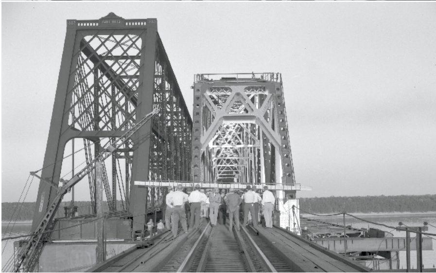
Bridge workers, IC brass, and even a dog were on hand as the first new span was moved into position on October 16, 1950. In this sequence, movement began at 9:30 a.m. (top), and by 10:08 the old span had been moved onto a temporary platform. The aerial view was taken in late morning. By 4:55 p.m. (above), the new span is almost in place, which occurred at 5:30. The bridge reopened to traffic soon after midnight.
