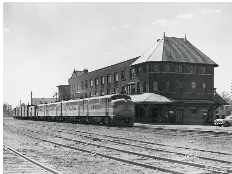
Outside Dixon's office in the landmark Middletown depot/headquarters building, four FT's amble past with an anemic three-car BC-3.
