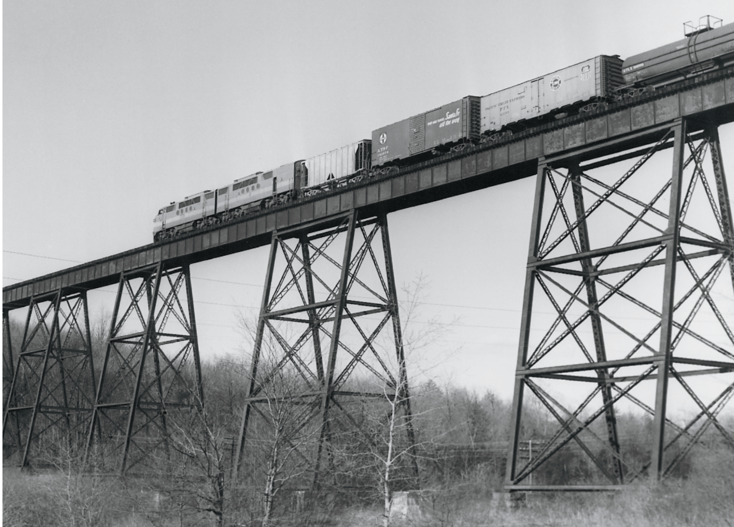
With my pal Roderick Craig, I followed train BC-3 of March 23 on its journey northwest from Middletown. About 38 miles out, the train flies over the 97-foot-high, 979-foot-long trestle at Ferndale, a structure emblematic of the tough, cross-valley course the O&W followed.
