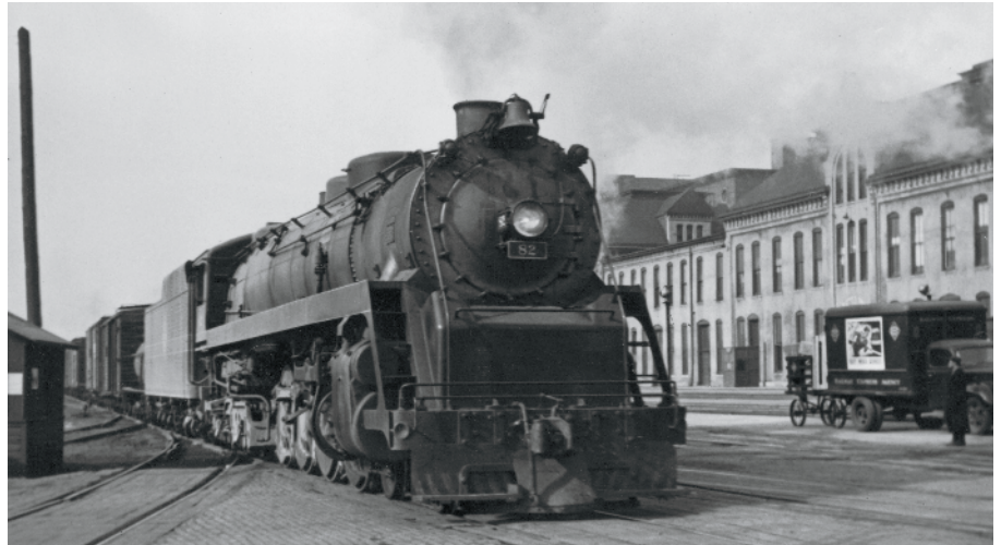
TP&W 4-8-4 No. 82 works east past Peoria & Pekin Union's Peoria Union Station in an undated photo during 82's 13-year career. The 1937 Alcos were among the lightest 4-8-4's.
