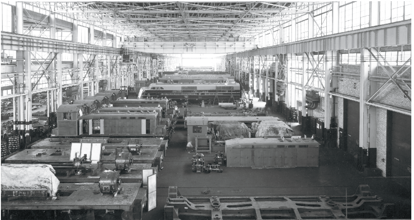
History takes shape at EMC's new La Grange plant in 1937. Beyond the switchers in the foreground, B&O EA No. 51 glistens in fresh paint.
