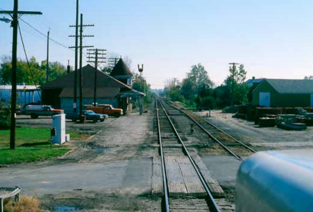
A 1977 view from the cab of an eastbound on the main track at Grinnell, Iowa, shows the siding situation there. Grades, road crossings, poor track, and a diamond crossing with a C&NW line (at the depot ahead) combined to make the 7,900-foot siding nearly useless for meets.
