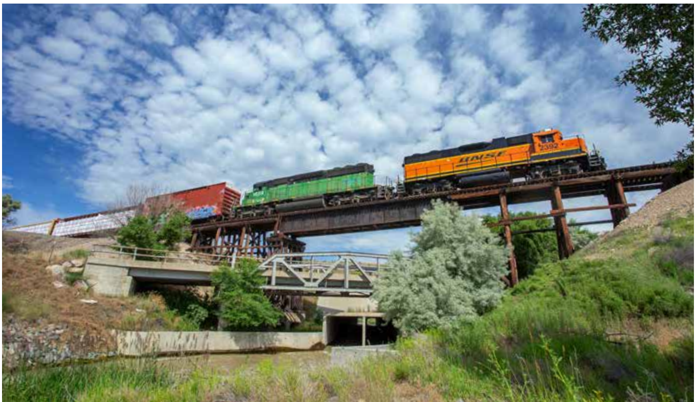
On June 28, 2018, GP38-3R No. 2392 leads former BN SD40-2 No. 1659 and the Cody Local across the old U.S. Highway 14 bridge and Alkali Creek Patch, in Ralston, Wyo. The faint initials of former owner CB&Q are visible on the bridge.
