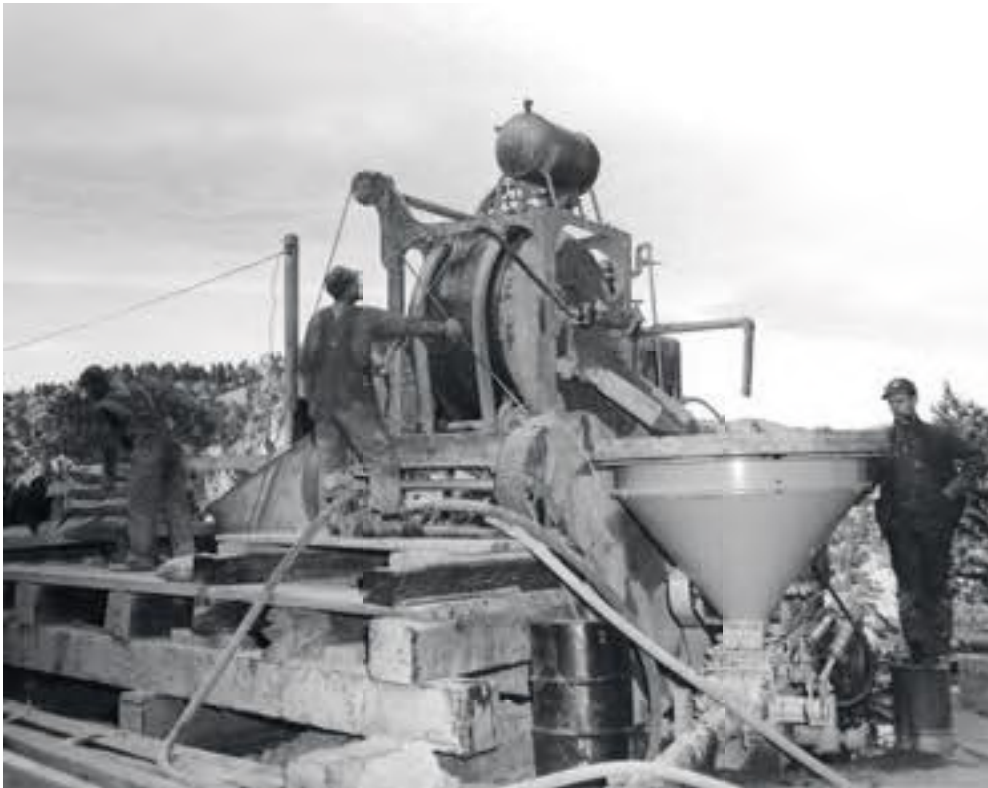
Concrete mixers mounted on improvised platforms (above) provided material for the tunnel's new lining. Portable generators (below) supplied electricity for the mixers and other equipment.
