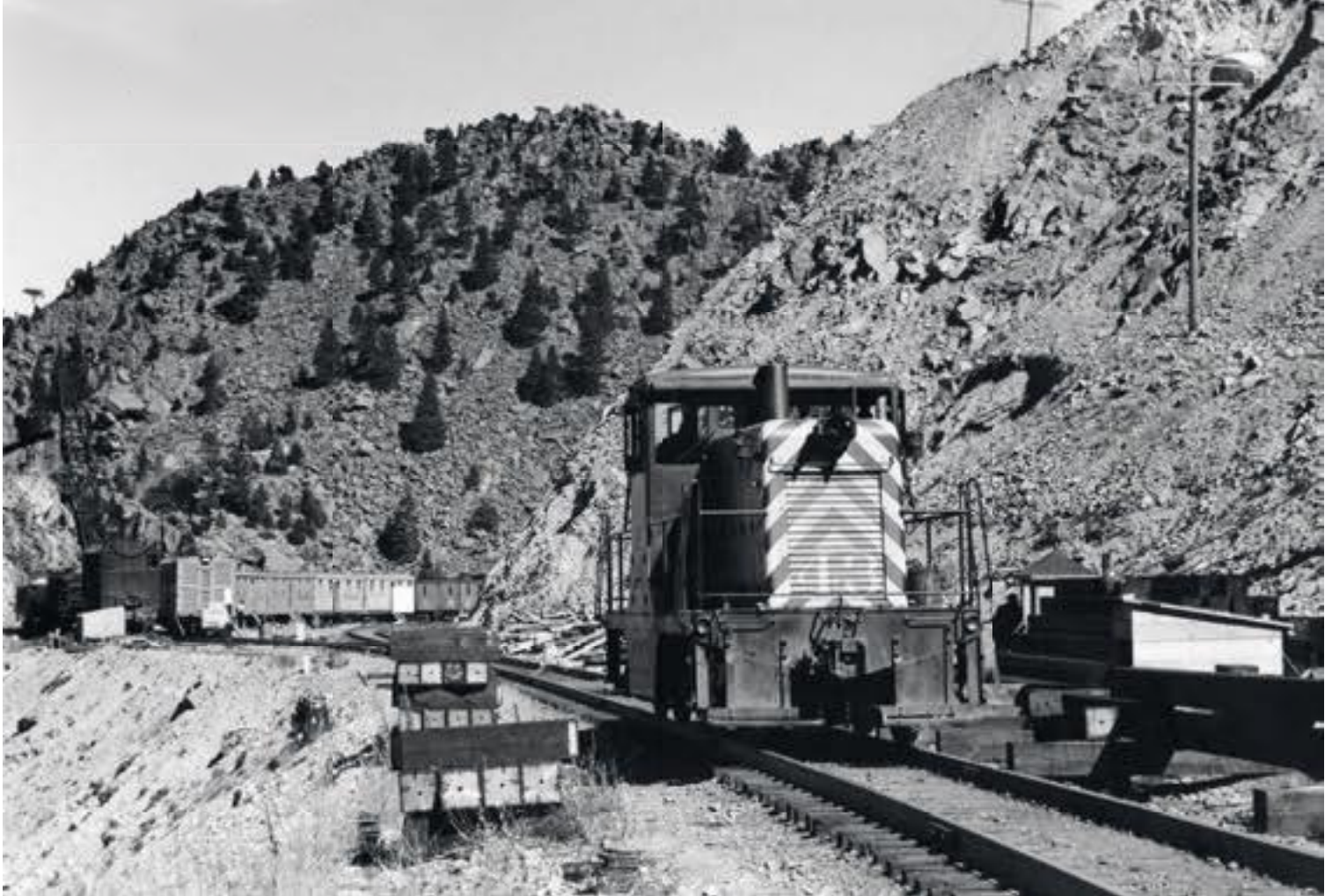
A Rio Grande GE 44-ton diesel shuttled equipment into and out of the tunnel. This view is east of the bore, where special tracks were built to accommodate outfit cars for workers.
