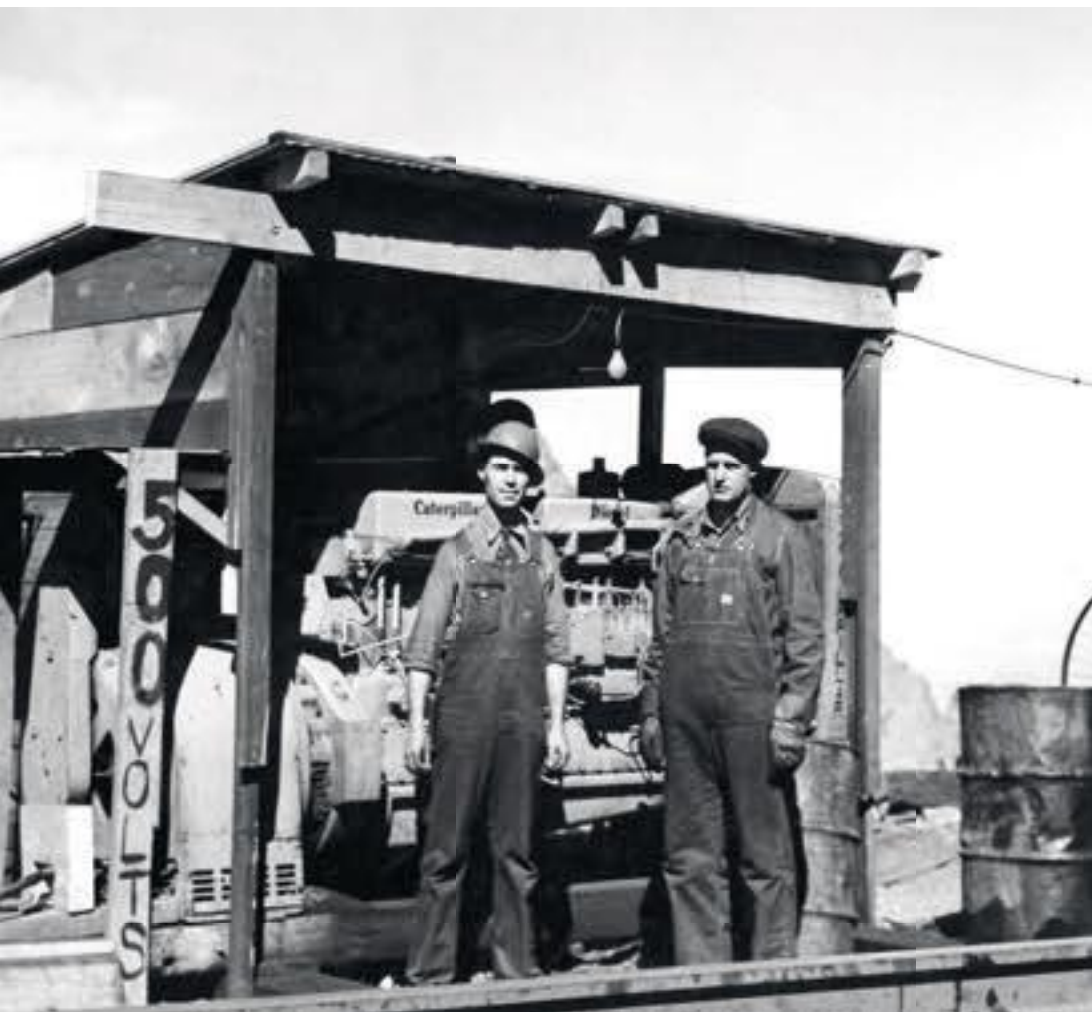
Concrete mixers mounted on improvised platforms (above) provided material for the tunnel's new lining. Portable generators (below) supplied electricity for the mixers and other equipment.
