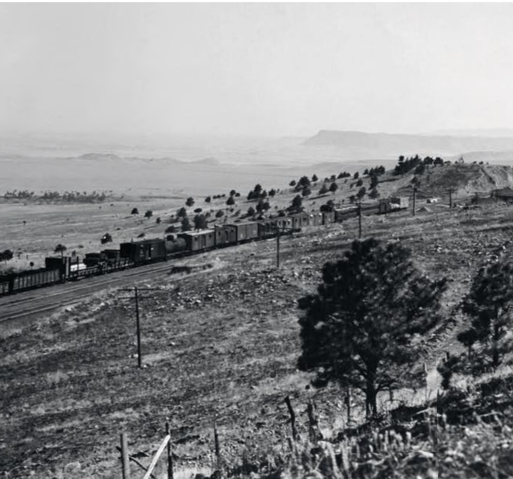
Plain, the first siding east of Tunnel 10 (a distance of 3 miles) became the headquarters for the men and equipment that repaired the burned-out bore. Perched on the edge of the Front Range, the location enjoys a sweeping view of the flatlands to the east.
