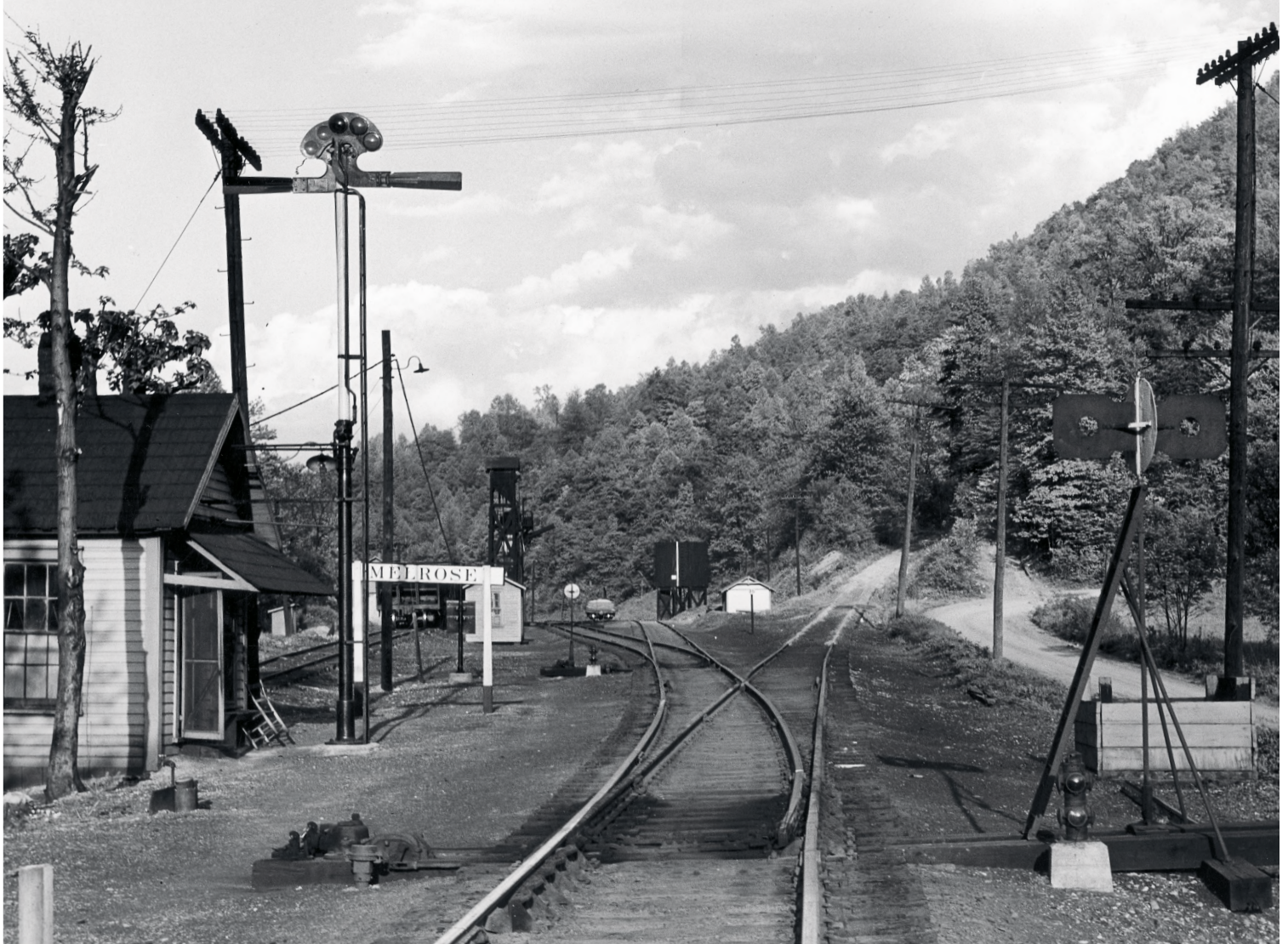
An eastward view at Melrose shows the extensive facilities at the base of Saluda Grade in April 1948. Around the left-hand bend beyond the water tower is Slaughter Pen Cut, where a carload of livestock perished in an 1893 runaway. The switch target for Safety Track No. 2 is mounted high for better visibility.
