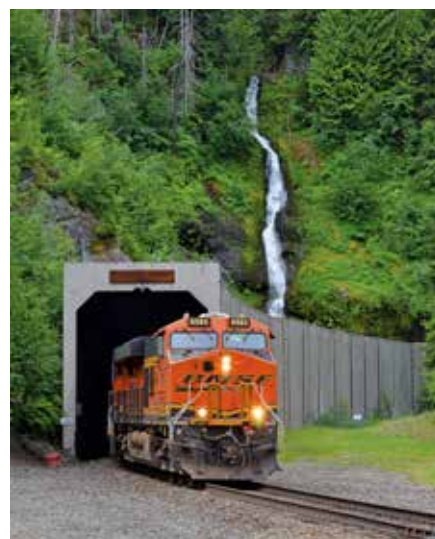
Empty grain train X-LVWTMP exits the concrete snow shed guarding the east portal of Stampede Tunnel at Martin. The grade will soon sharpen to 2.2 percent on the descent to Easton. Bruce Kelly
