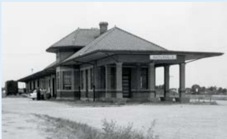
The station at Gatesville, Texas, most soundly constructed and beautiful on the system, marks the west end of the Cotton Belt.
