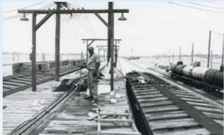
Laborers top off the bunkers of refrigerator cars at the Pine Bluff icing platform, one of two on the Cotton Belt system.
