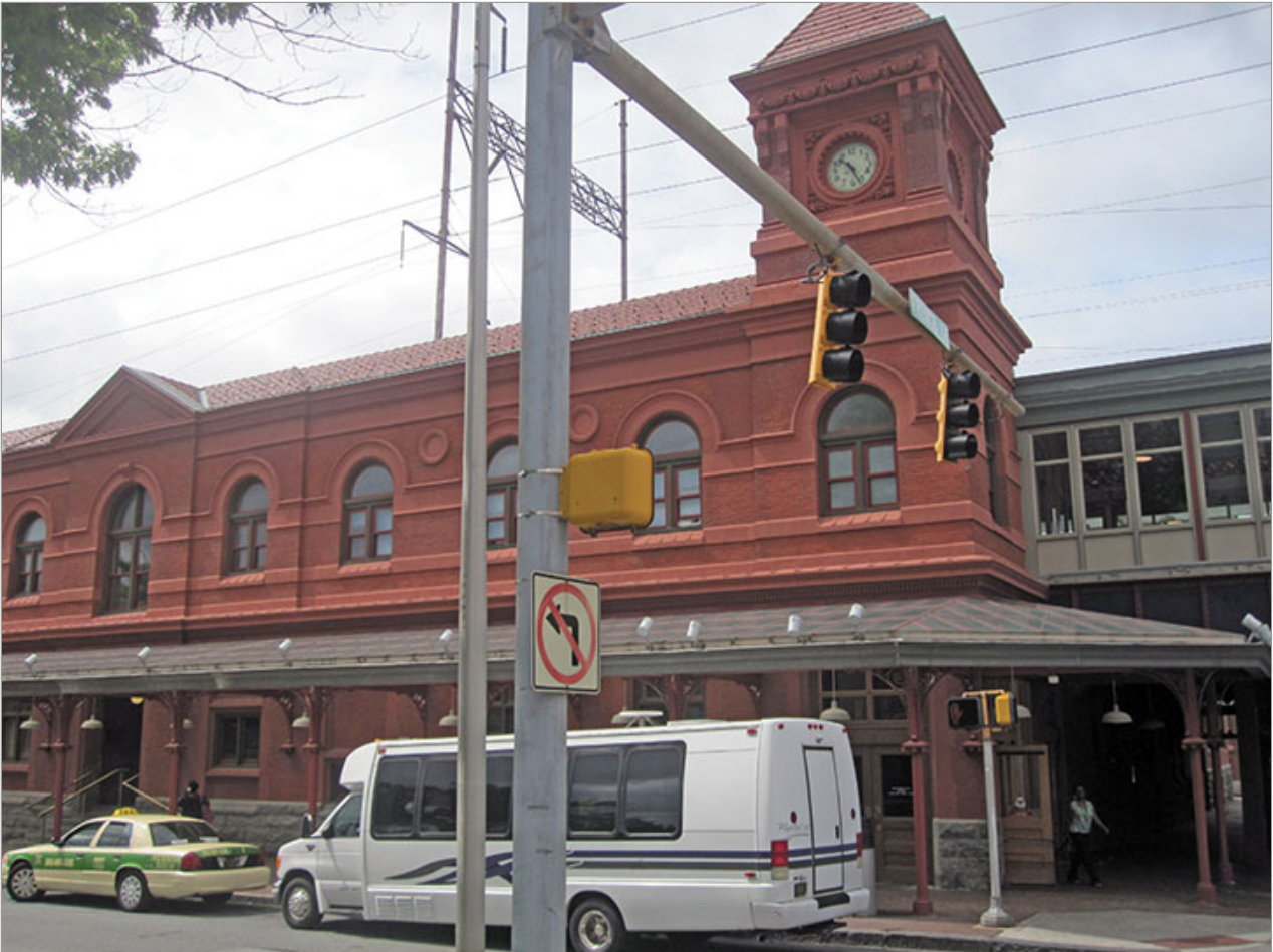
The beautifully renovated Wilmington station—now also known as the Joseph R. Biden Jr. Station—is shown in 2015.
