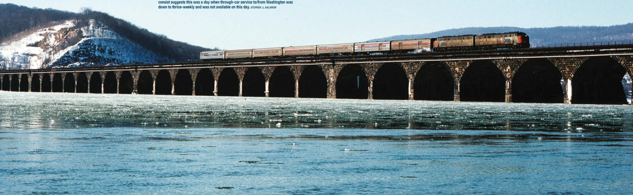
A pair of gritty E-units eases across famous Rockville (Pa.) Bridge on Feb. 4, 1978, west of Harrisburg. Completed in 1902, the famous bridge remains the longest stone-arch railroad viaduct in the world. It crosses the Susquehanna River about five miles north of Harrisburg and is still used by Amtrak's Pennsylvanian . The short consist suggests this was a day when through-car service to/from Washington was down to thrice-weekly and was not available on this day. STEPHEN J. SALAMON
