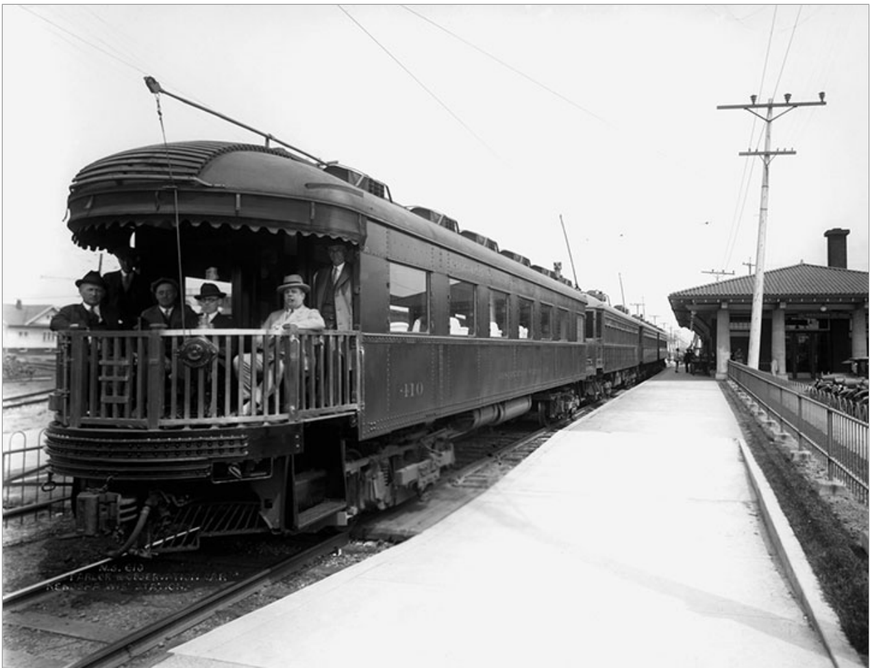
A morning northbound Limited replete with a parlor-observation car pauses at the Kenosha, Wis., station circa 1925. The Prairie House-style depot designed by Arthur Gerber, typical of so many on Insull-controlled Chicago interurbans, still stands. North Shore photo, Krambles-Peterson archive.
