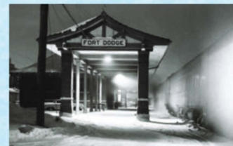
LEFT Activity is sparse at IC's pagoda-style station in Fort Dodge as the Hawkeye awaits departure. In the good 'ol days, this is where the Omaha section of the Hawkeye was separated from the Sioux City section.
