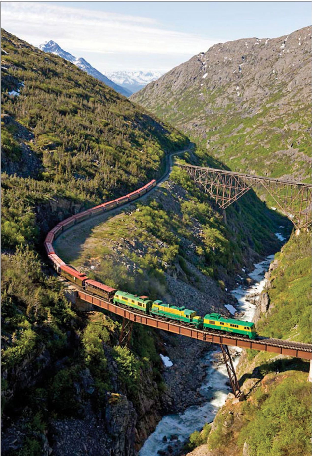
The cantilever bridge at Mile 18.6 was bypassed in a 1969 line relocation that also necessitated the railway's second tunnel. The original steel span
