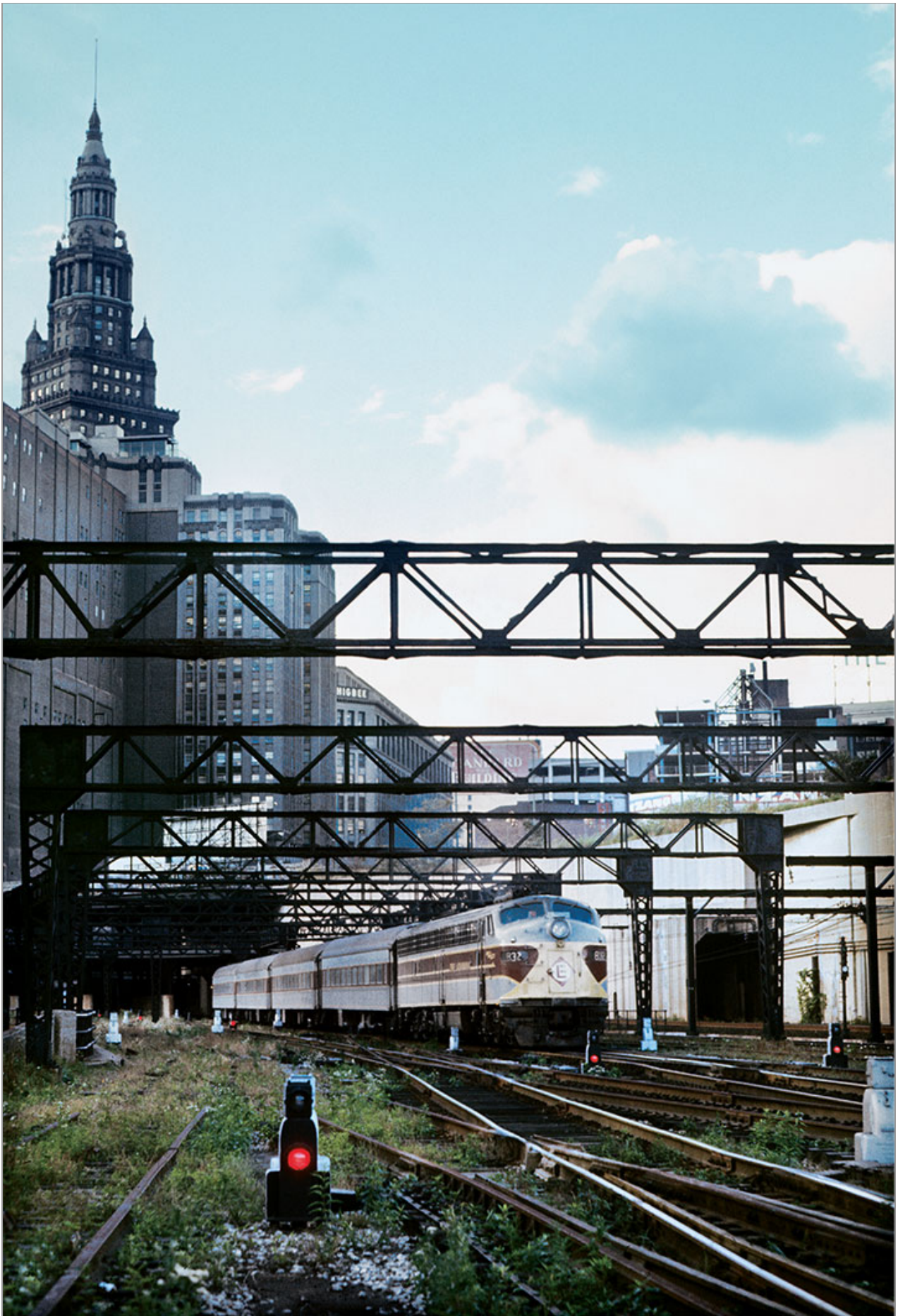
The sun is setting behind the buildings of downtown Cleveland as train 28 rolls forth from the bowels of Terminal Tower (background), for years the
