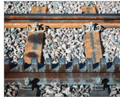
ABOVE: This photo taken at the Manitou Springs station shows the difference between the more traditional outside rail and the cog rail in the middle, which helps propel the train uphill. JUSTIN FRANZ PHOTO
