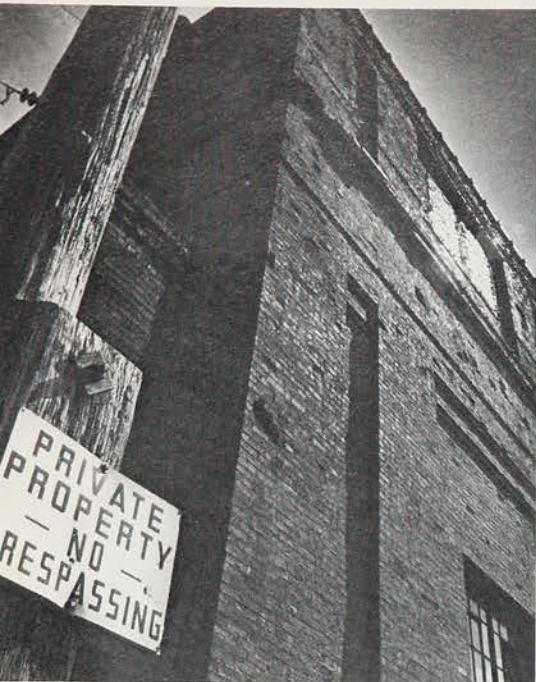
SUBSTATION FACADE, May 1978.
