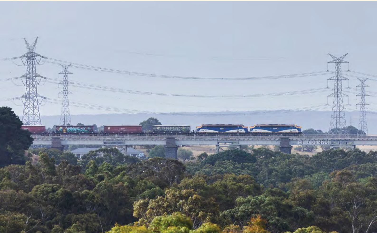
Above: Nearing its destination, the B class led train is seen later in the afternoon of Sunday 12 February crossing the Moorabool viaduct near Batesford, on the steady descent from Warrenheip to Geelong. Scott Gould
