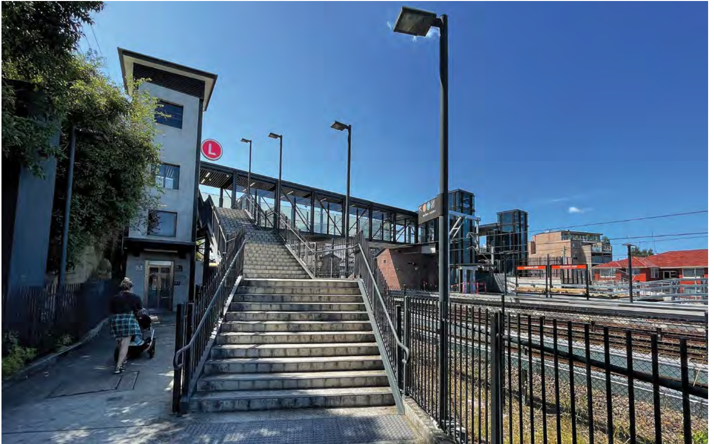
Above: The stairs and lift linking Dulwich Hill Station with the adjacent L1 light rail terminus (behind the photographer). The new footbridge shown in this view has enabled a more direct connection between the two modes, whereas previously pedestrians had to loop round via Bedford Lane and Wardell Road. The stairs (and photographer) are on the spot once occupied by the east fork junction points between the former branch from Rozelle/Darling Harbour and the Goods Line still visible in the right hand foreground. The L1 light rail route now occupies the bulk of the former branch right-of-way, except for the triangle junction's former west fork, which sits abandoned about 200 metres to the south (or right) of this view.
