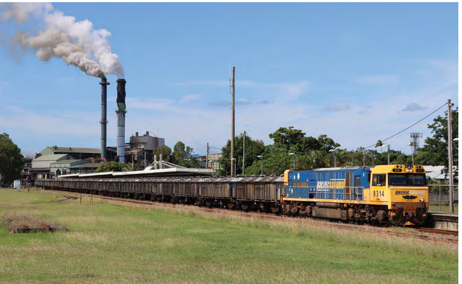
Below: On Sunday 8 January 2023 Proserpine Sugar Mill is still crushing into the new year as PN unit 8314 leads Proserpine to Mackay Harbour loaded sugar train 6ZP6 past the station so that the mill siding points can be reset for the North Coast Line before departure. Luke Horniblow
