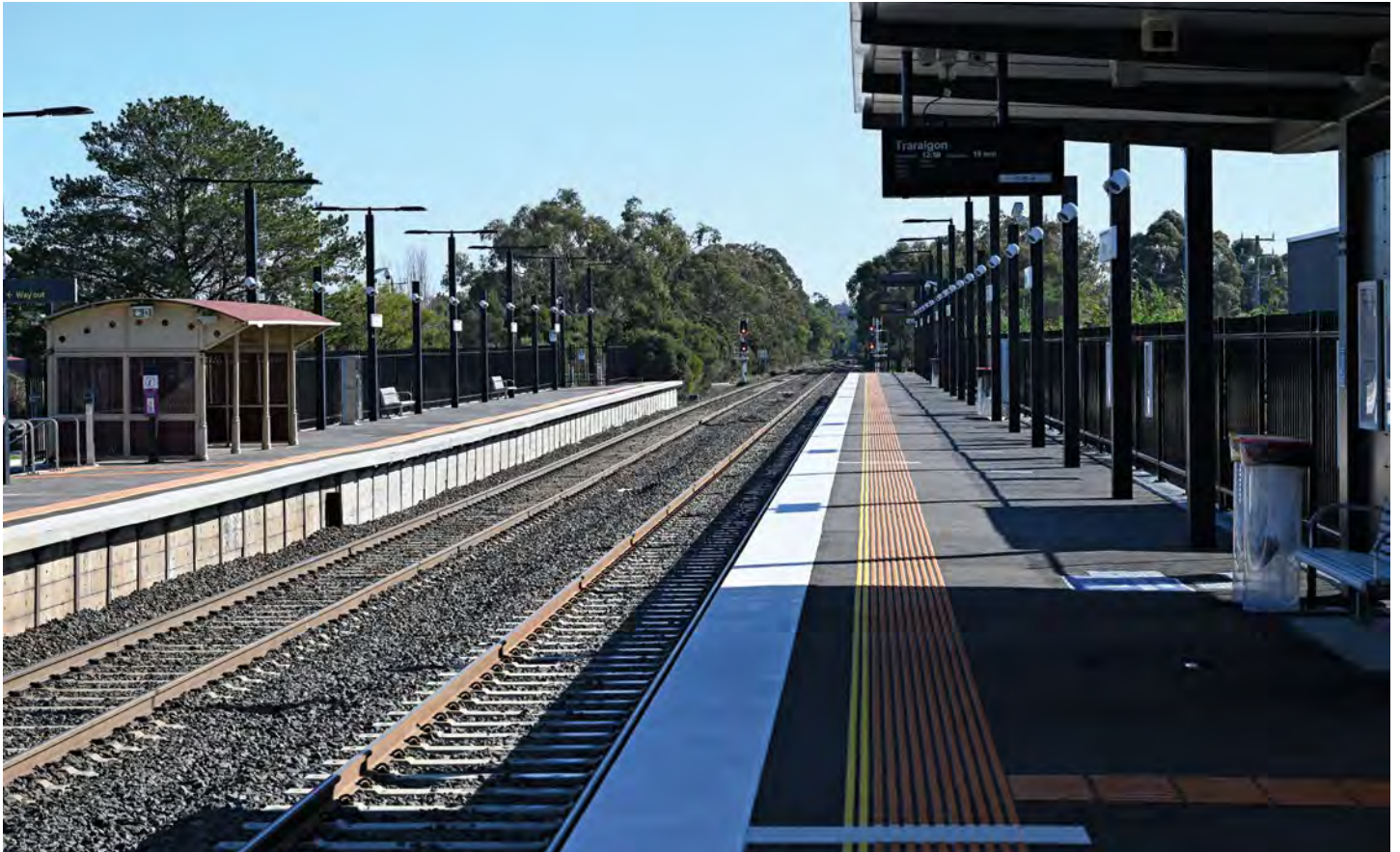
Looking in an Up direction from the new platform at Longwarry, the track extension through the platform before the single line commences is evident. A few hundred metres beyond the signals, the double line reverts to a single line about where the shadow across the track is seen.
