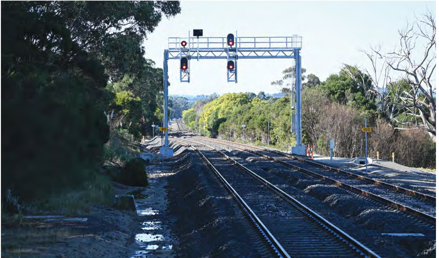
Looking in the Down direction from Bunyip station, the two lines negotiate a few curves before forming the single line towards Longwarry. The visible curve boards (yellow pointy ended signs with black numerals) require trains to slow, however in practise most trains stop at Bunyip, so few trains have to slow down for these curves.
